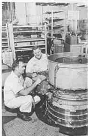
HORIZONTAL hoist which goes 10 feet into the ground holds engine which is being rebuilt by overhaul mechanics Neal Smith and Sherm Grant, right.
